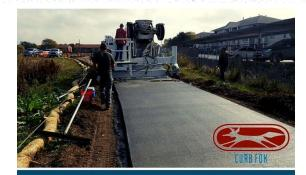
CONCRETE PAVING MACHINE
